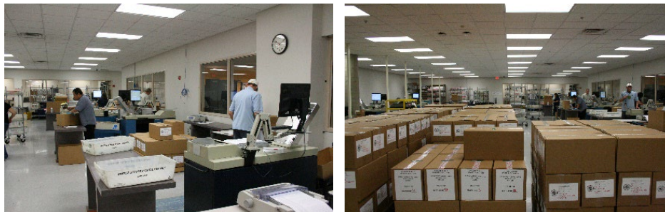
Ballot Tabulation Counting (BTC) Center: Pre-General Election 2020 Photo with ballots stored in BTC under sprinklers
