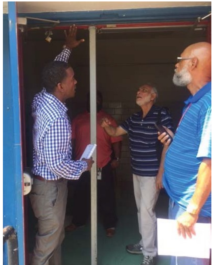
BOE, DGS and ODR staff members work to remove the astragal (center pole) from the polling place doorway to meet accessibility standards.
