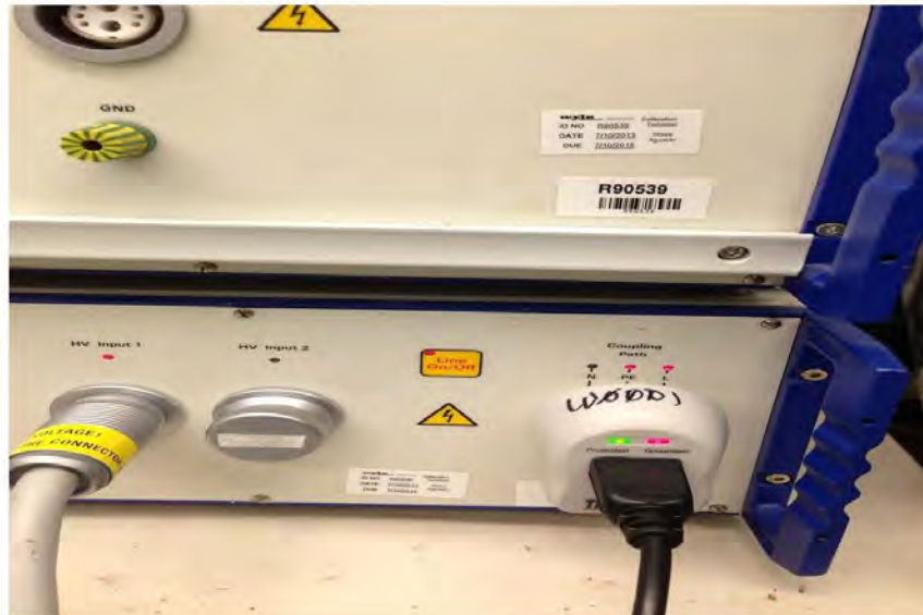
Photograph 12: ES&S FL EVS 4.5.0.0 Lightning Surge
