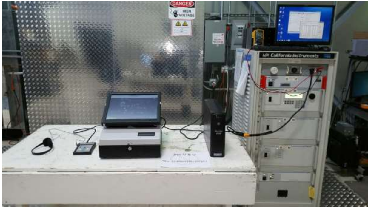
Electrical Power Disturbance Test Configuration Photograph - OVI-VC
